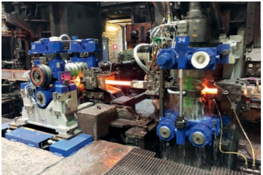
The new Red Ring Series 5 rolling stands will enable Stahlwerk Annahütte to reduce roll-change times. They are also easier to operate.
