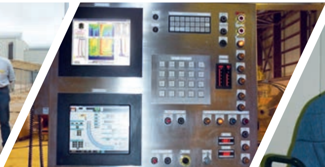
The Mold Expert HMI, neatly embedded into an operator station casting-platform pulpit
