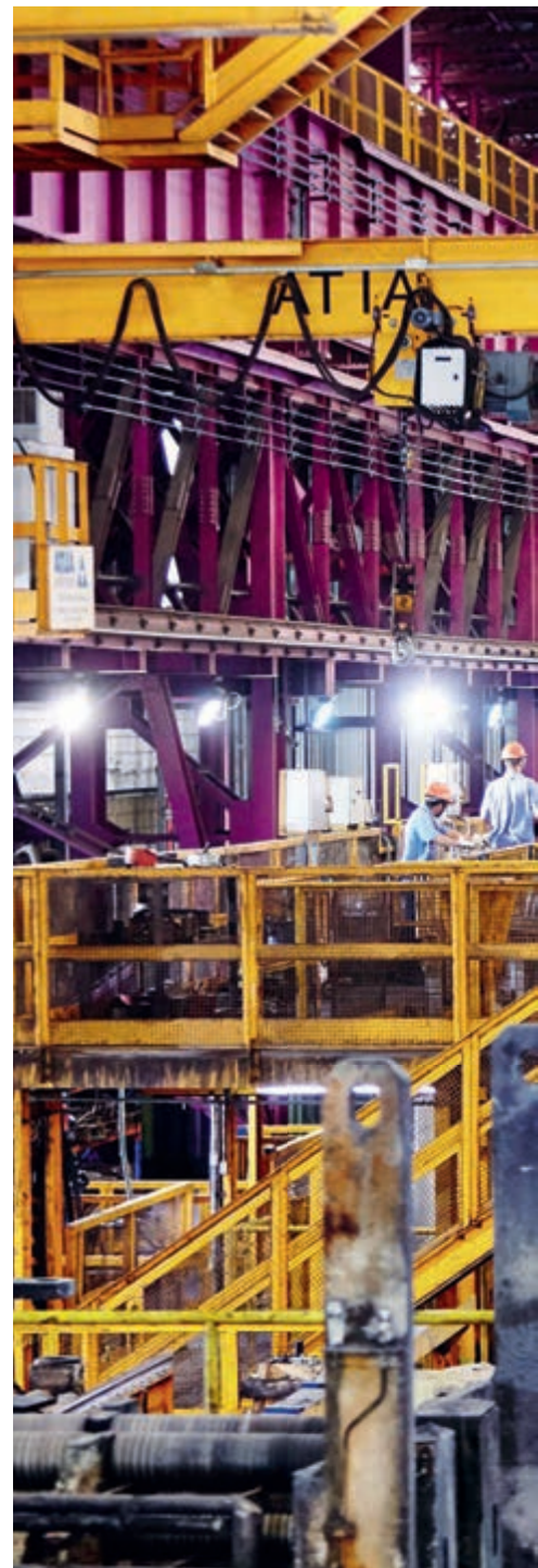
FIG. 1: MAT provides actionable information whenever needed—and enables steel producers to increase efficiency in maintenance.
