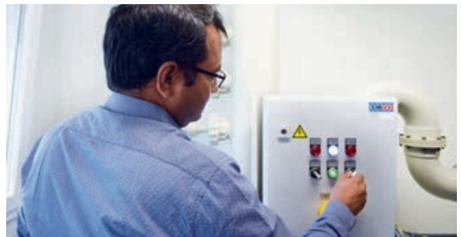
FIG. 2: In order to comply with environmental standards, the simulator only works if the acid-fumes cleaner is turned on.
