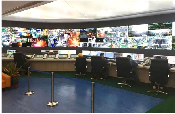
Figure 4 - Operation Control Center, China
